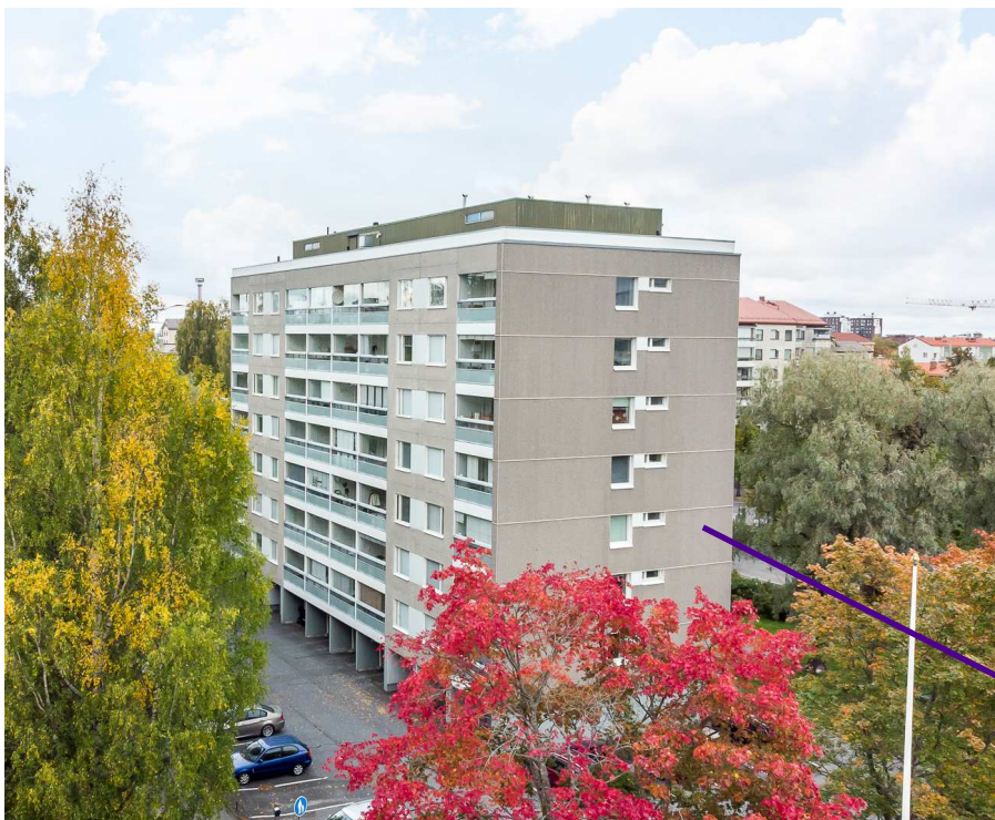
Image source: https://www.annelkv.fi/tampere-amuri-kerrostalo-5/
